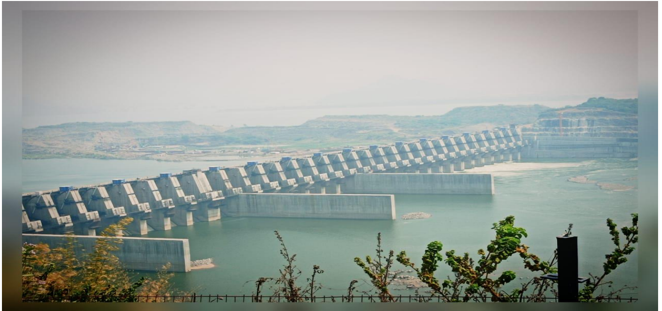
CONSTRUCTION SITE VIEW OF POLAVARAM PROJECT
